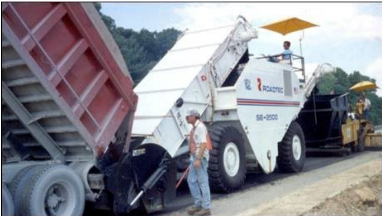
Figure 13.24-2. Material Transfer Device
