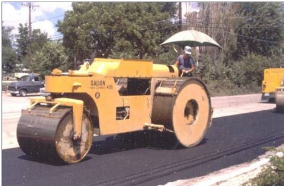
Figure 13.24-6. Three Wheeled Roller
