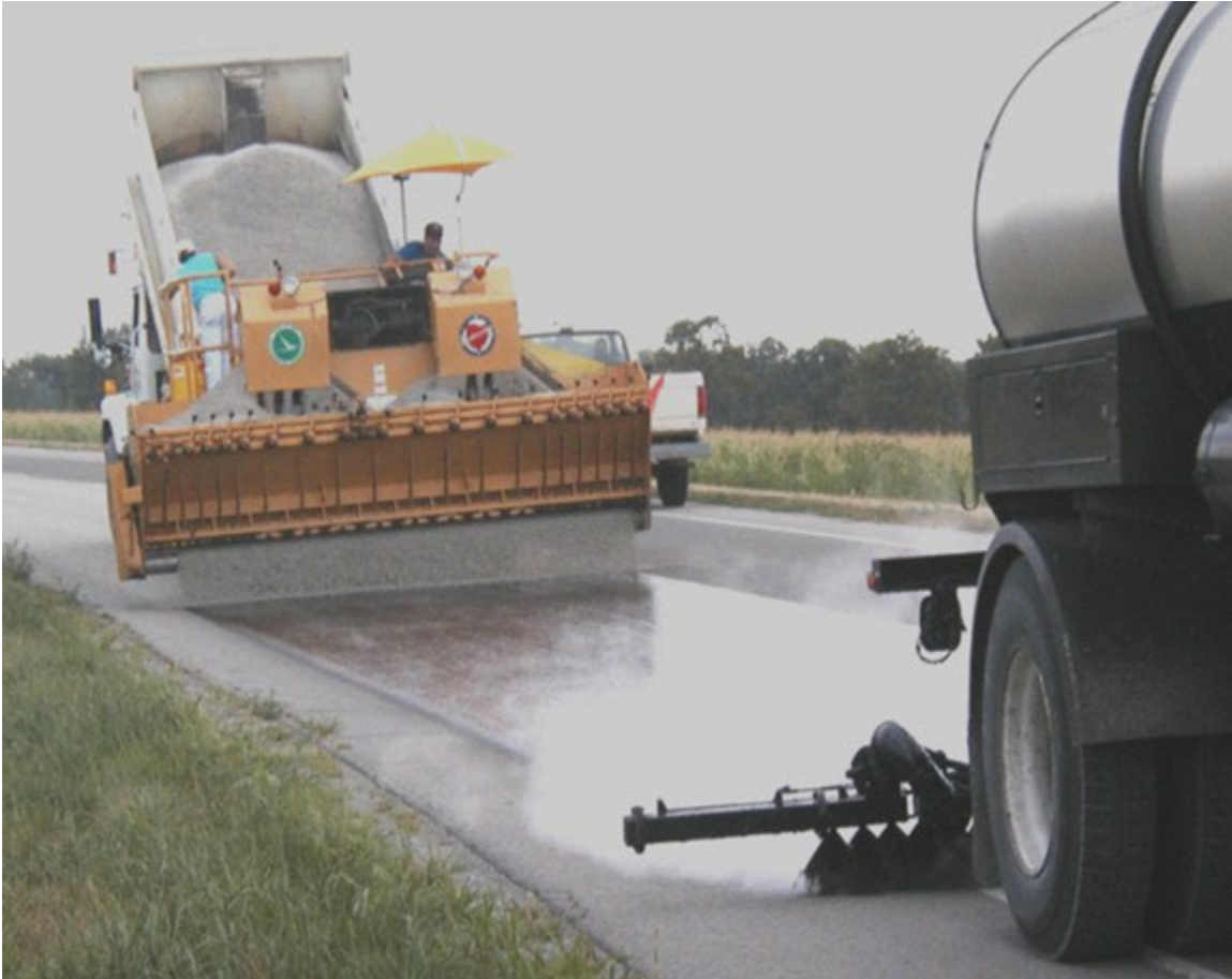
Figure 13.24-11. Aggregate Spreader
